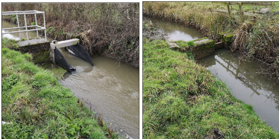
Figure 3.1-5. A tilting weir (left) and stop-board weir (right) within the Gwent Levels. Water control (or penning) levels are managed by the Internal Drainage District, with higher control levels during the summer for local water availability, and lower control levels during the winter to reduce flood risk.
