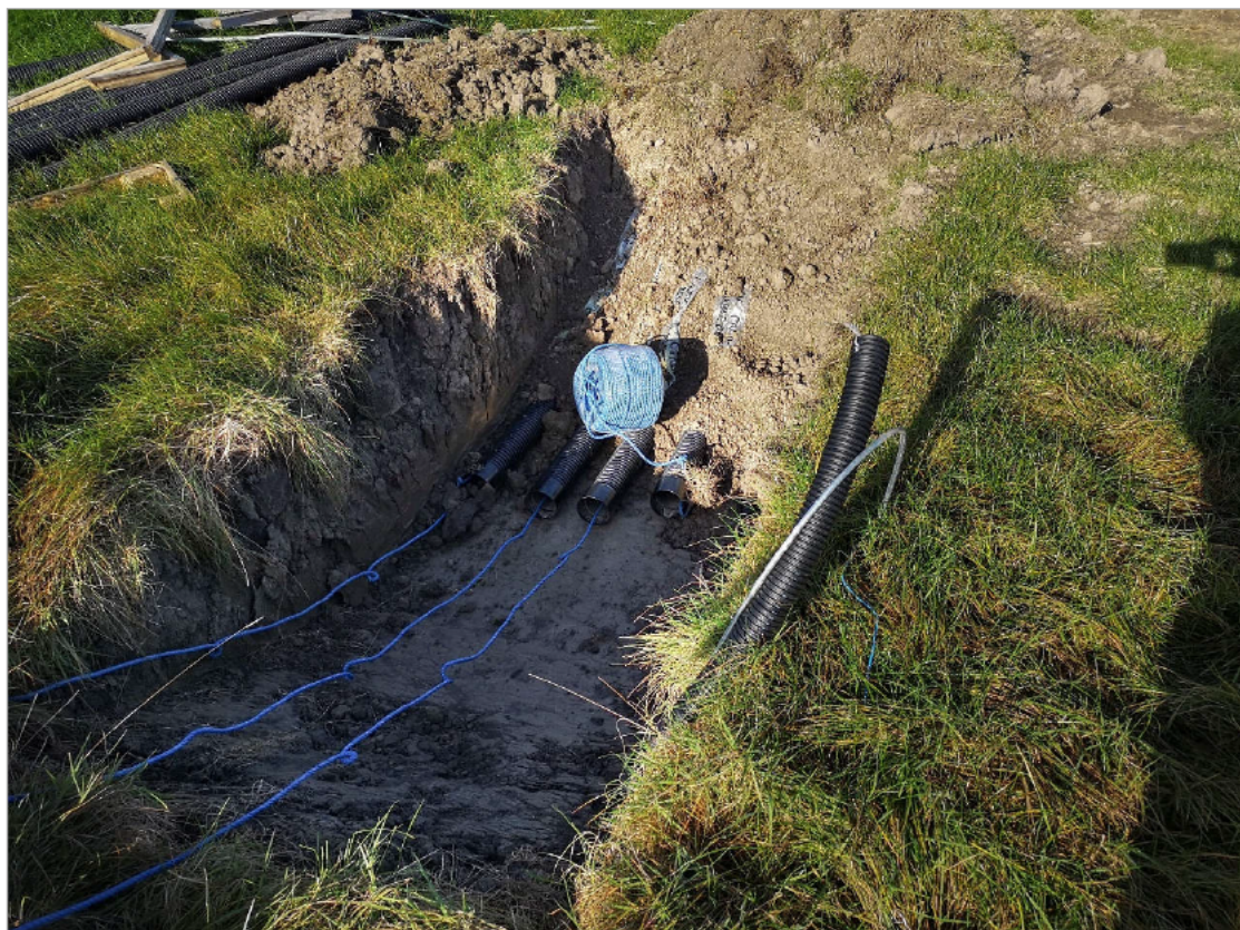
Figure 3.2-3. Photograph of a cable trench during the construction phase of the Llanwern solar farm. The black cable duct tubes can be seen in the backfilled trench; the blue ropes are for pulling the cables through the ducts.
