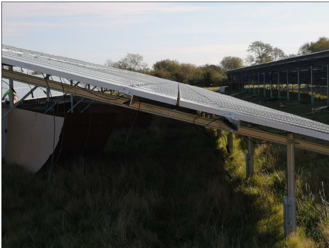
Figure 3.2-1. Photograph showing solar panel arrays at the Llanwern solar farm, which was under construction at the time of writing. The 25 mm gaps between the panels can be seen at centre, and the supporting posts at bottom-right.
